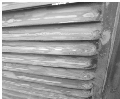
Fill and sand hood louver repair area
